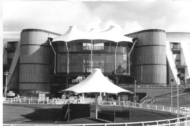
designer Nigel Browne says. "Fabric can achieve far greater spans than conventional roof materials, with minimal supporting structure. For the roof to the Saddle Bar on the link building, a fabric structure was the obvious solution.
